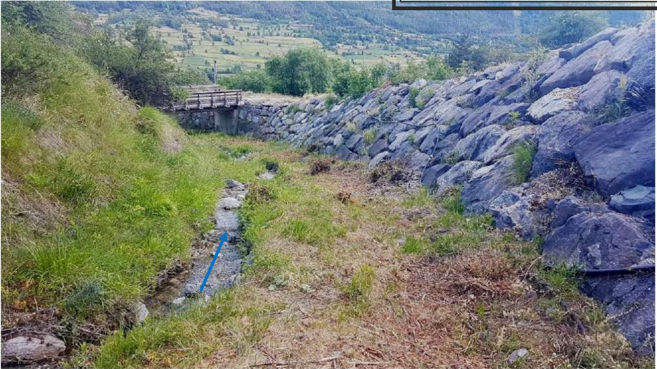
Figure 106: Pont du Rif Claret
